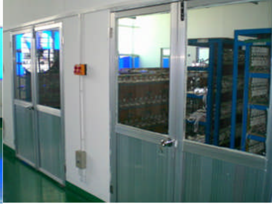
Aging test room 2
